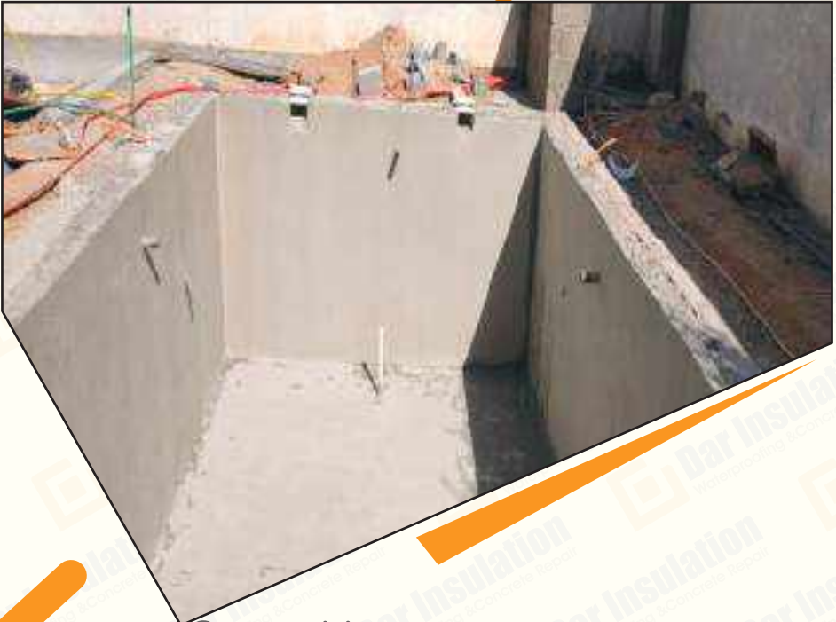
Cementitious Waterproofing For Swimming Pool
