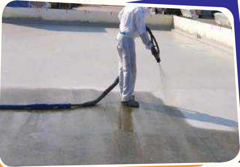
Polyurea For Roof Deck
