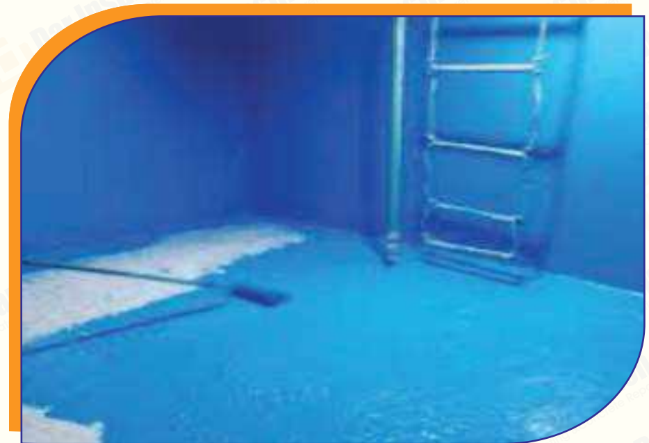
Epoxy Coating For Internal Water Tank
