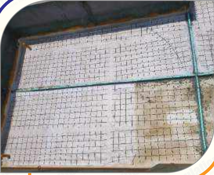
Expansion Joint Screed
