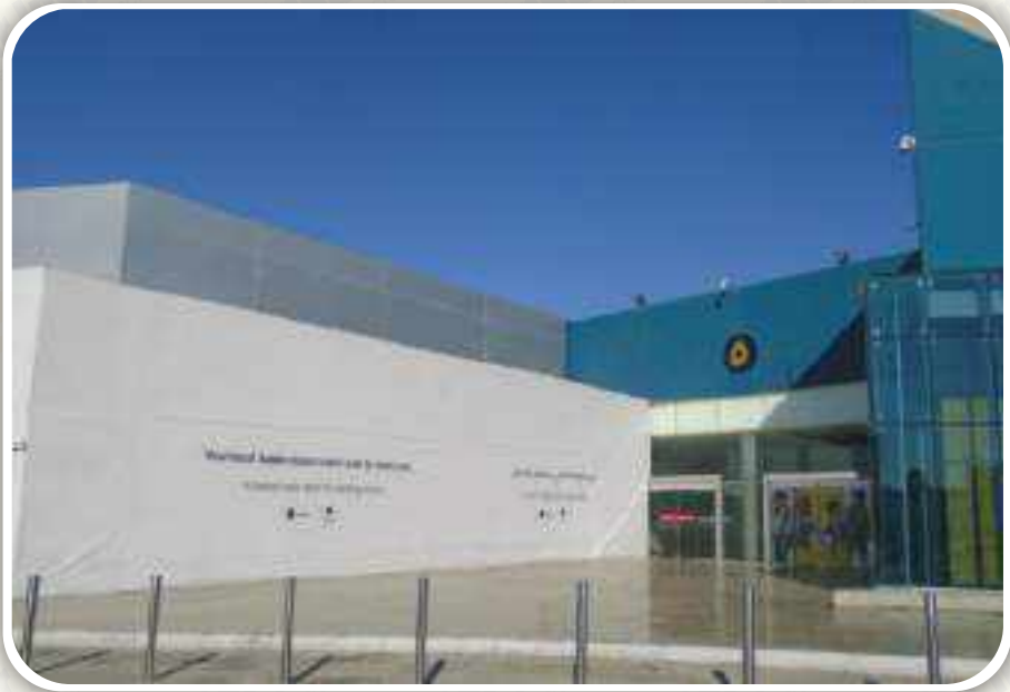
DHAHRAN MALL GATE 5 ROOF WATERPROOFING
