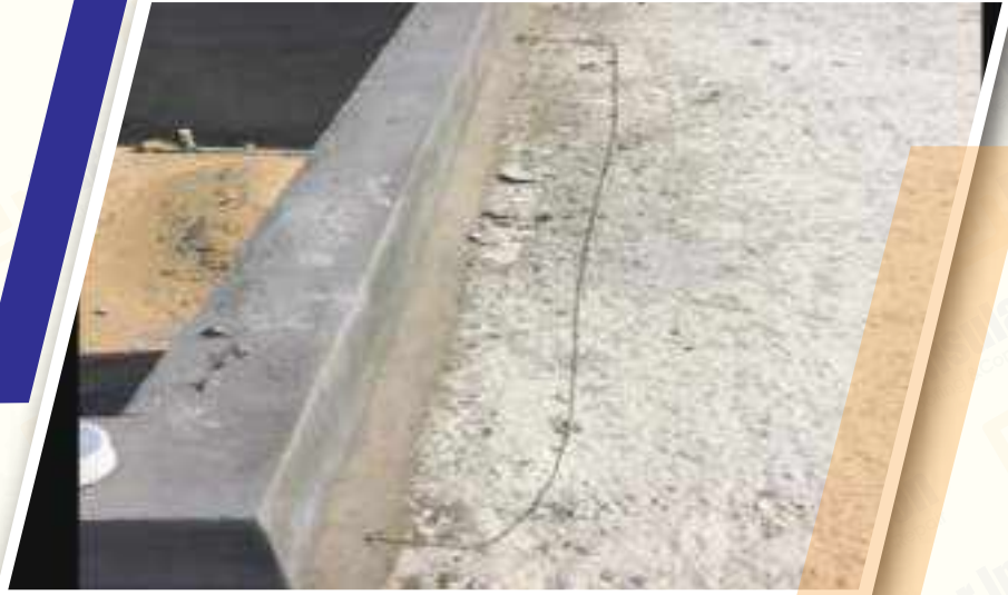
CANT STRIP MORTAR 45 DEGREE
