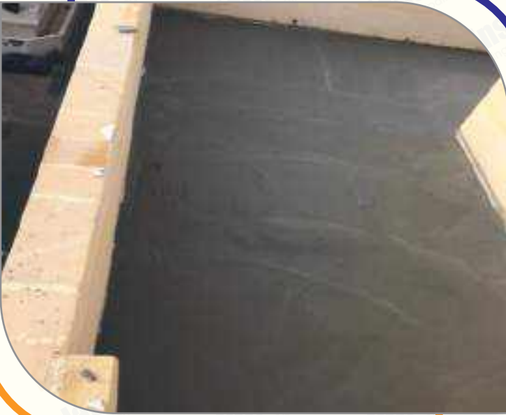
Concrete Finish Helicopter
