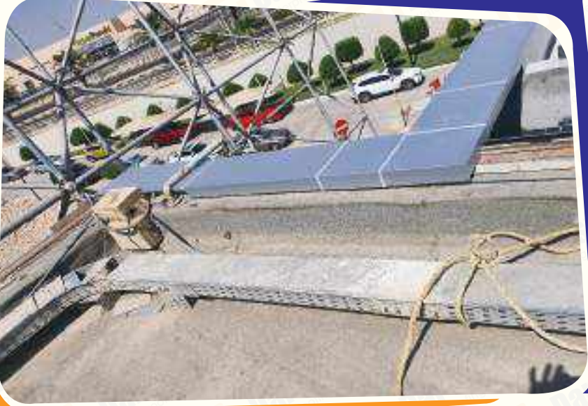
Expansion joint treatment
