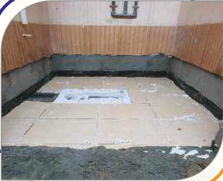
Wet Area Waterproofing
