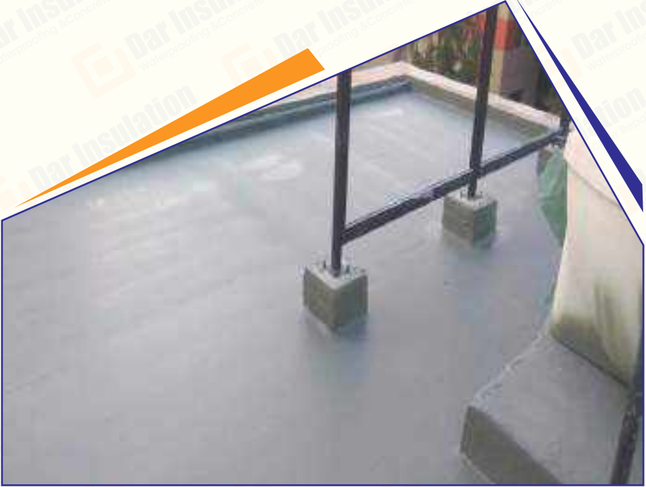
Polyurea For Roof Deck
