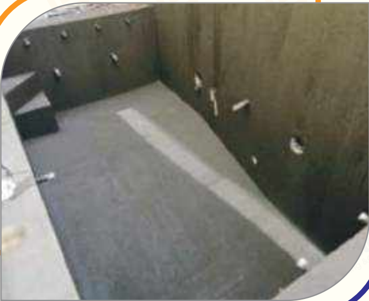
Cementitious Waterproofing For Swimming Pool
