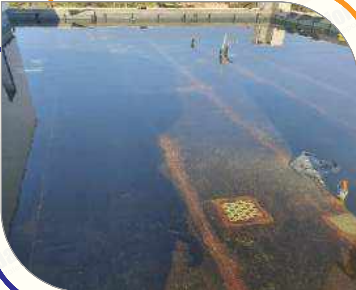
Bituminous Waterproofing Membrane Water Test
