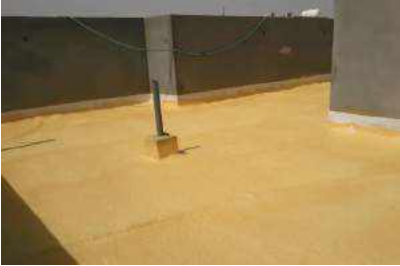
POLYURETHANE FOAM SPRAY
